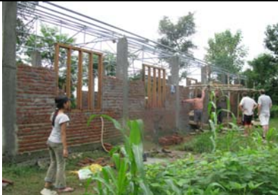
Building build by volunteers
