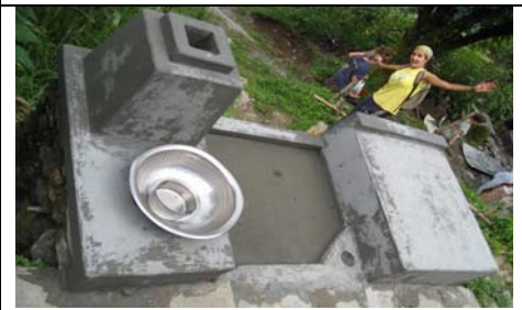
Soak pit build by volunteers
