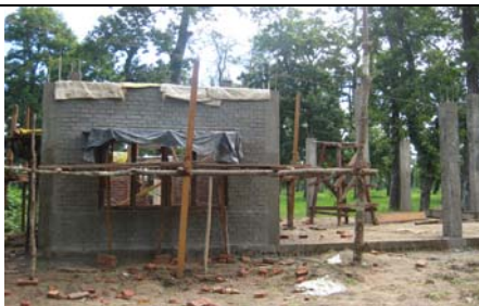
Newly build building by volunteers
