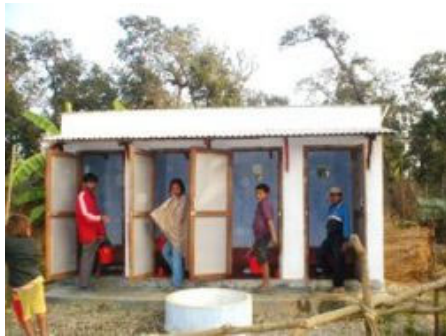
Toilet construction October 2005, Ujjwalnager, Chitwan
