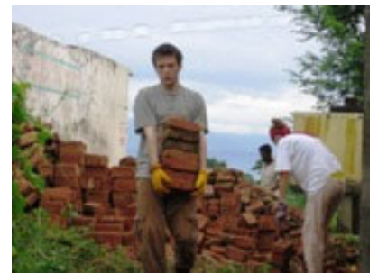
Volunteers carrying bricks for building the classrooms
