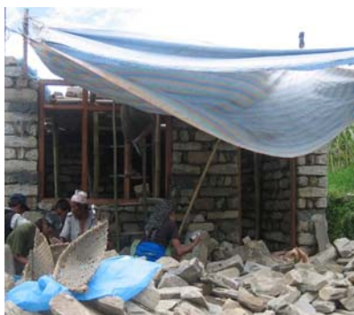
Under construction community center
