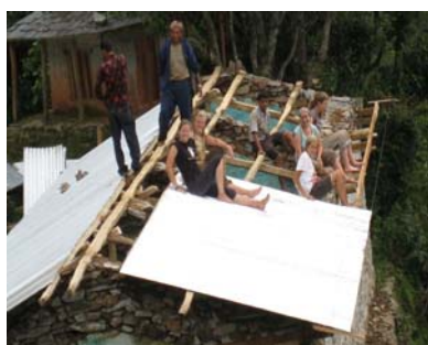
Under construction building
