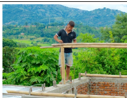
Phase III – Figure 4. Construction bamboo roof structure and villagers fixing bamboo in place
