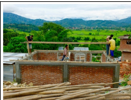
Phase III – Figure 4. Construction bamboo roof structure and villagers fixing bamboo in place
