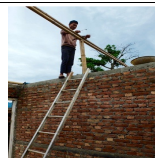
Phase III – Figure 4. Construction bamboo roof structure and villagers fixing bamboo in place
